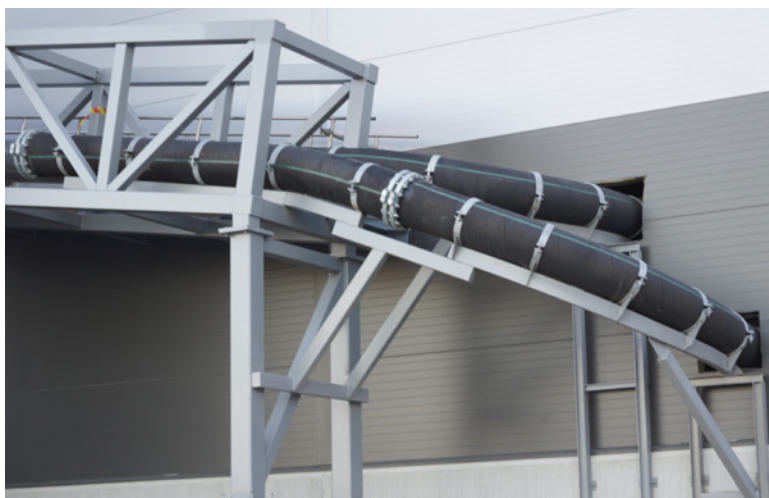
Picture 5: Swivel Hoses used to exit concentrator (tailing line and serial pumping).
