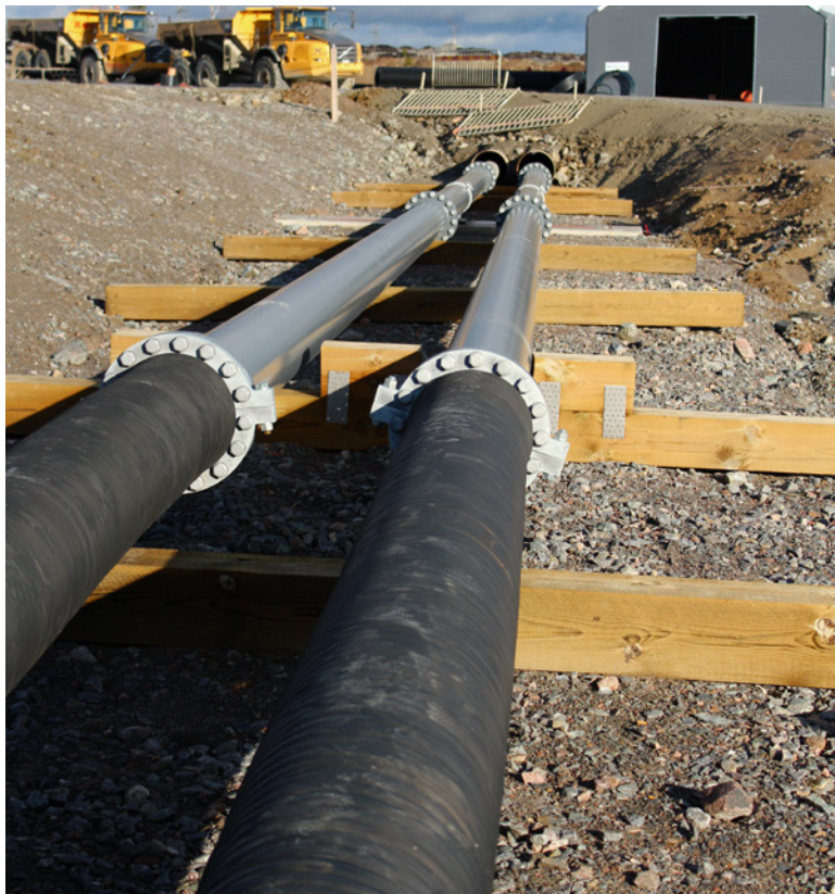
Picture 4: Tailing Line with Swivel Hoses and Rubber lined steel pipes.
