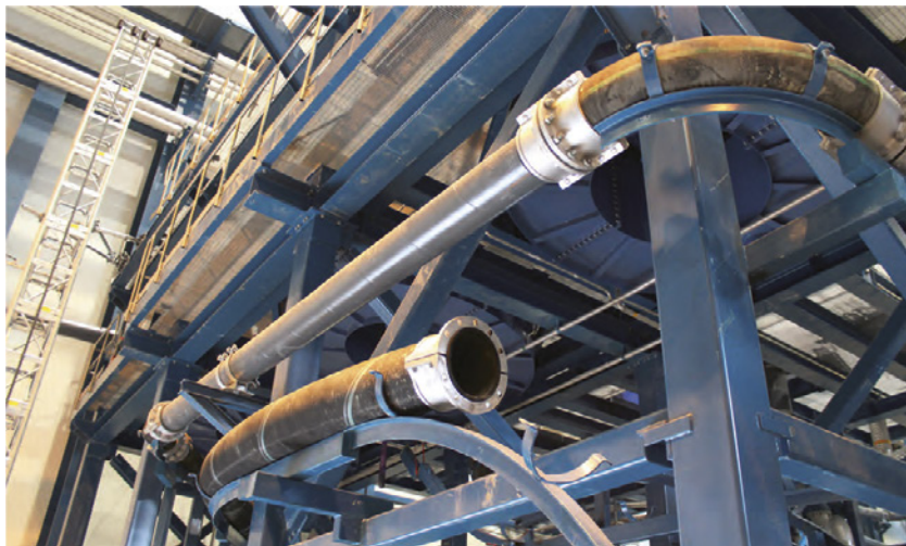
Picture 3: Material handling hose, rubber lined steel pipe, 3xD 90 Degree bend and support clamps
