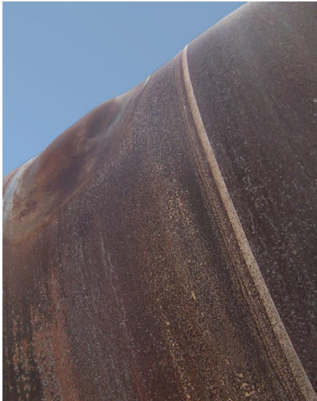
Shell profile (or out-of-roundness) is a permanent deformation of the kiln shell. This is normally referred to as shell blisters, shell warp-age, shell twisting, or coke bottling.
