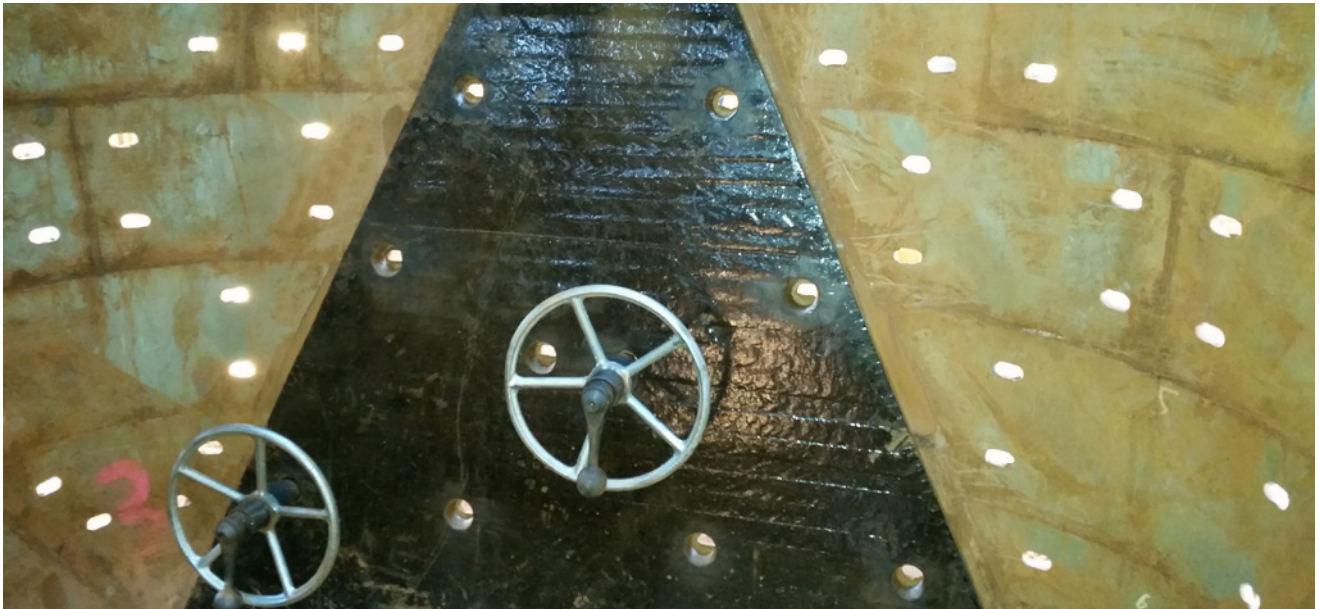
SafeFit clamps holding a liner in position awaiting the installation of Taper-T attachments.
